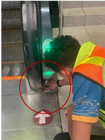
Figure 4. Manual Operation of Escalator (Source: Author documentation, 2024)
